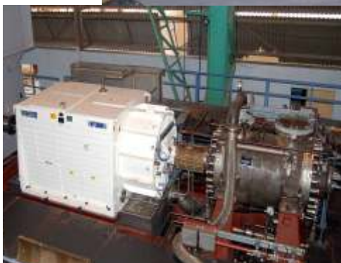
String test of natural gas compressor driven by job motor for Marmul, Oman
